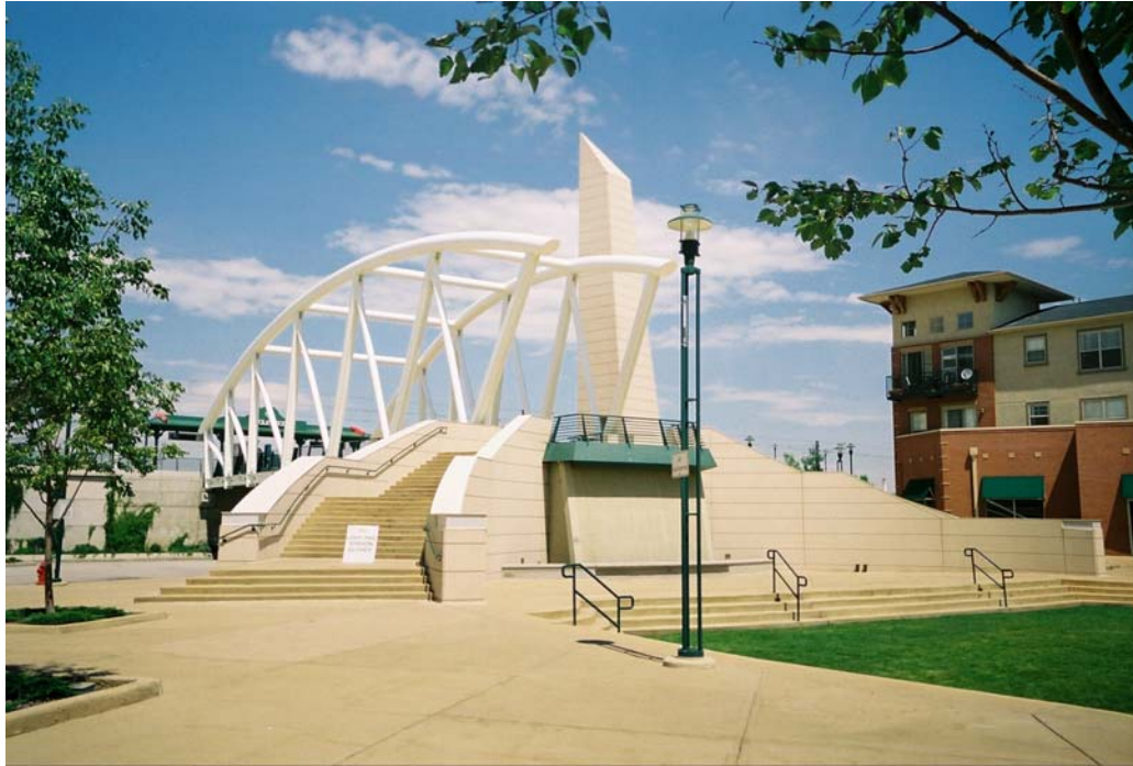
City of Englewood, Colorado, Transit-Oriented Village, light rail station. This is a mixed-use development that contains a civic center, retail, office and apartments.
