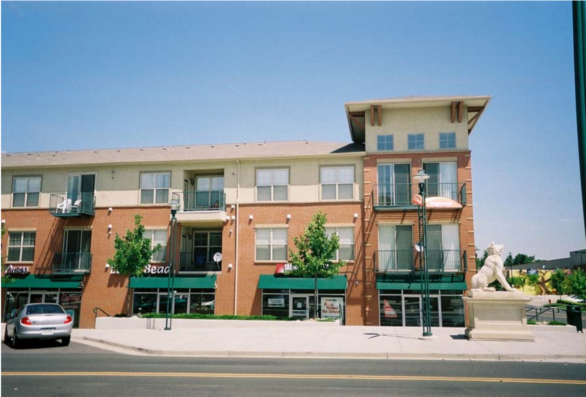
Englewood City Center TOD mixed use development, retail on first floor and apartments on the upper stories.
