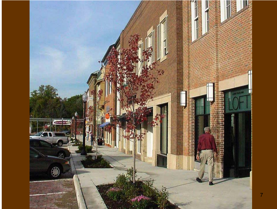
City of Hudson, First & Main new mixed-use development
