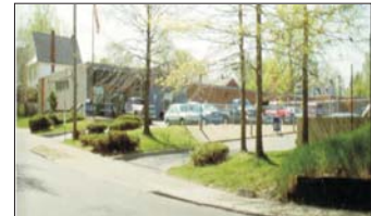
The current East Cleveland Post Office is smaller in square footage, parking spaces, and acreage than post offices that have recently been built in Greater Cleveland.
