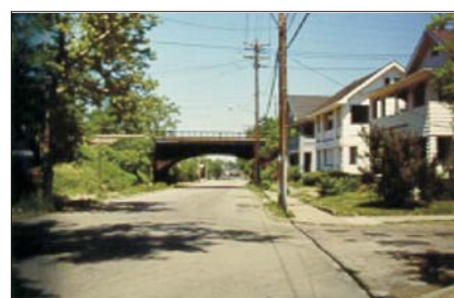
Collamer Street, looking northwest from Elderwood Avenue. Proposed street closing at railroad overpass
