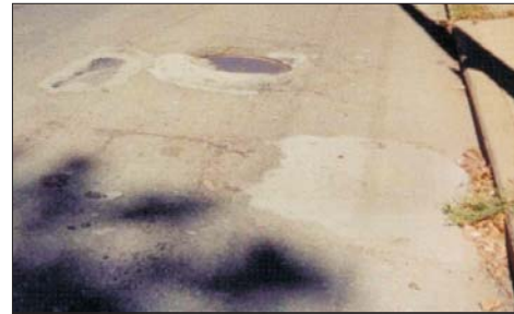
Deteriorated Pavement.
