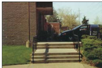
The steep site requires steps to reach the entrance, which limits access for persons with disabilities.
