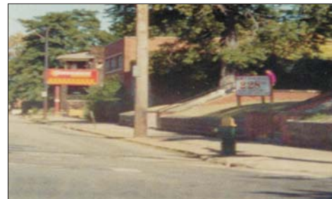
Curb of Inadequate Height.
