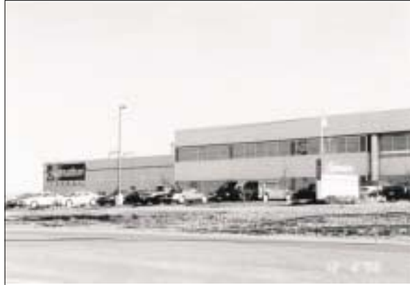
The 432,000 square foot Mr. Coffee/Sunbeam building, which opened in 1997, is the largest development to occur in recent history in the Village. Over 56% of the Village is currently zoned for industry.
