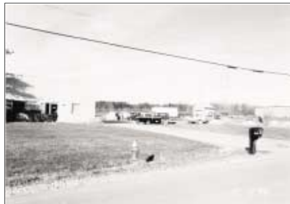
The lack of landscaping and screening of outdoor storage on many properties along Bond Street detracts from the appearance of the area and harms the image of the Village.
