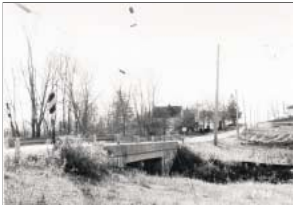
The Cochran Road bridge over Beaver Meadow's Creek has been identified in poor condition. Replacement or major repair of the bridge would be an ideal time for building a covered bridge which could act as a gateway to the center of town.
