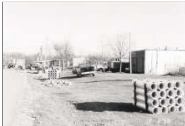
The poor performance of residential and industrial septic systems is effecting water quality in Tinkers Creek. New sewers are needed to alleviate this problem and allow new development.
