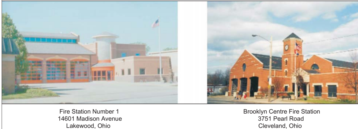
Exhibit 5-6. Examples of Fire Stations
