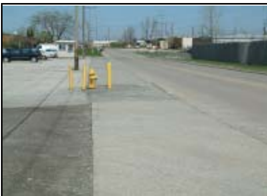
Parking lots fronting roadways which lack defined entrances present dangers for drivers and pedestrians.
