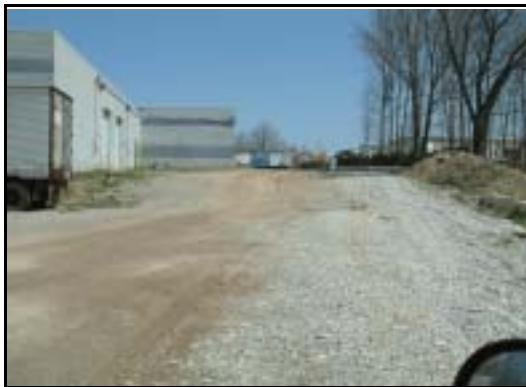
Access drives and parking lots lacking improved surfaces are unstable and present drainage problems.
