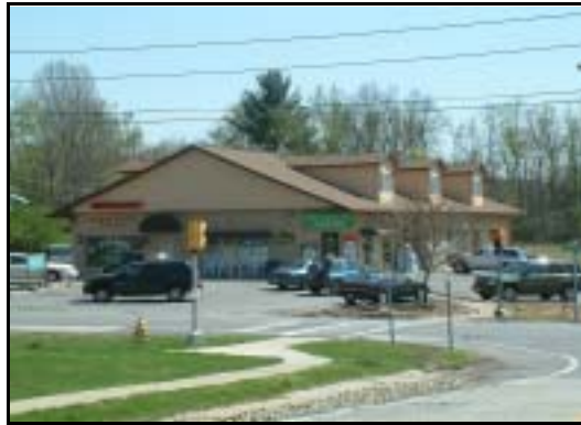
Commercial retail building at the Village Center.
