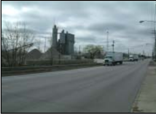
Northfield Road entrance from Bedford (east side).
