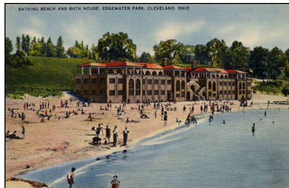
Figure 2-21: Historic Bathhouse at Edgewater Park Source: The Cleveland Memory Project
