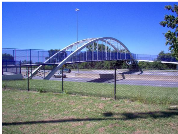
Figure 2-27: Gordon Park Pedestrian Bridge 39
