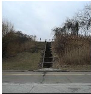
Walkway off Ramp - North
