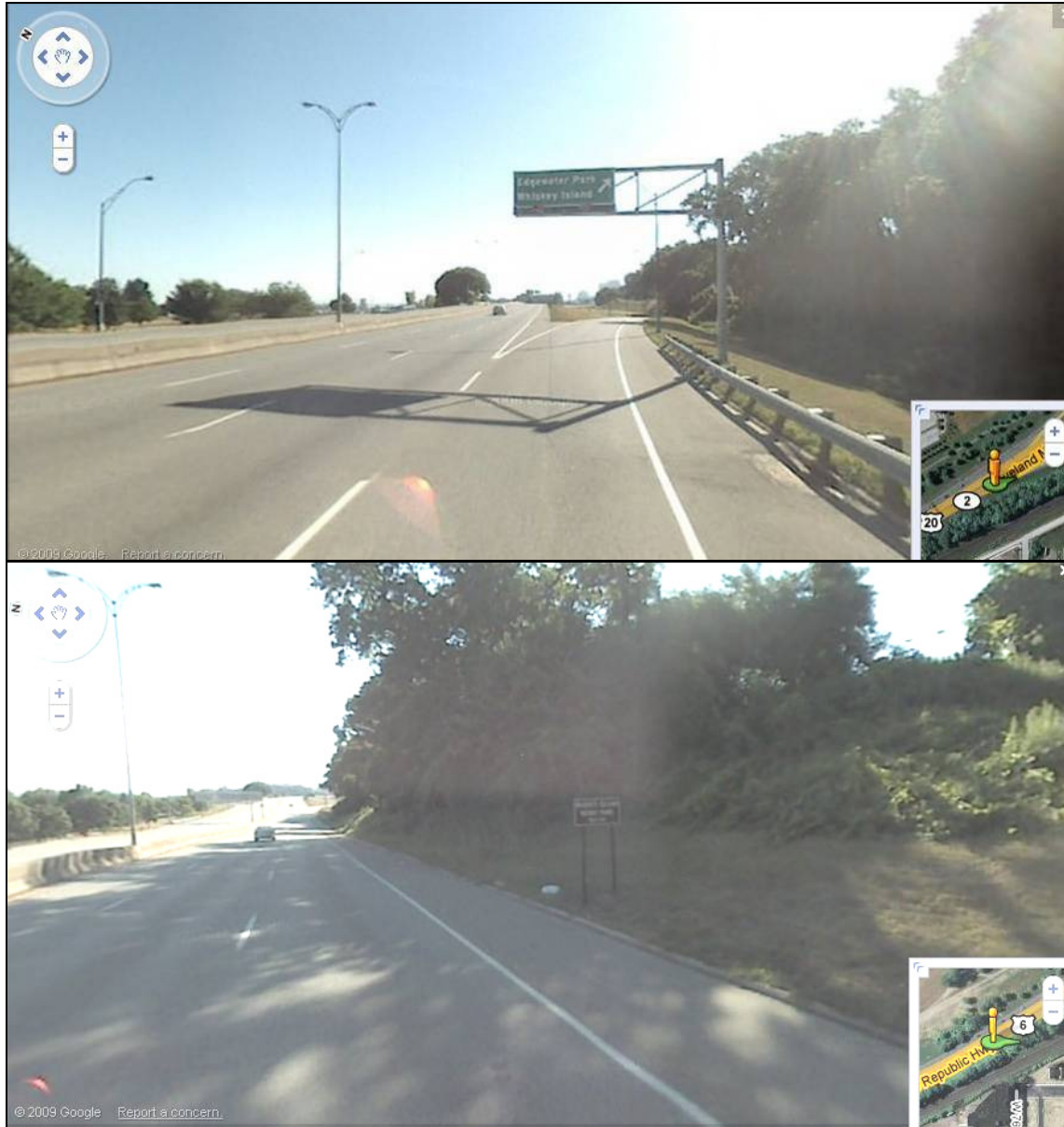
Figure 3-13: West Shoreway Exit Ramp to Edgewater Park Source: Google Maps
