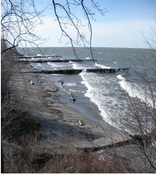
Figure 5-2: Perkins Beach looking west
