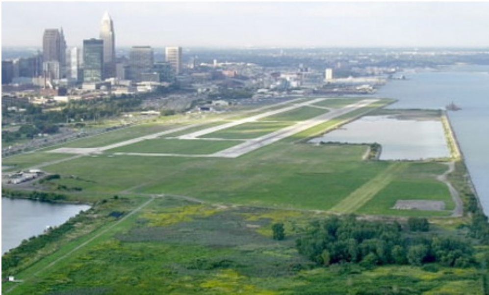
Figure 5-27: Photo of Burke Lakefront Airport. 35
