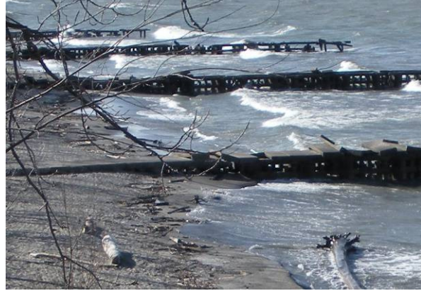
Figure 5-3: Perkins Beach groins
