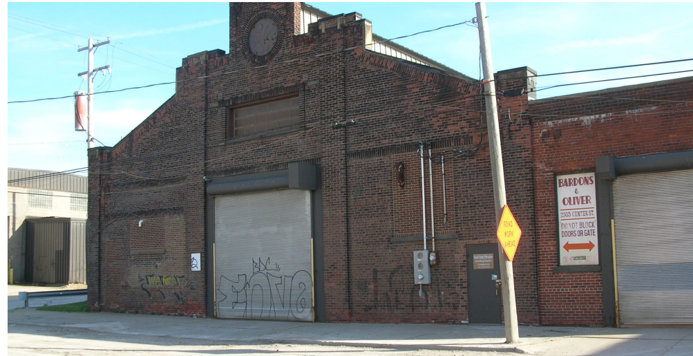
FIGURE III.27 - SOUTHWEST CORNER OF CENTER AND HEMLOCK; BRICK STRUCTURE WITH GABLE ROOF, ROOF MONITOR AND CLERESTORY LIGHTING.
