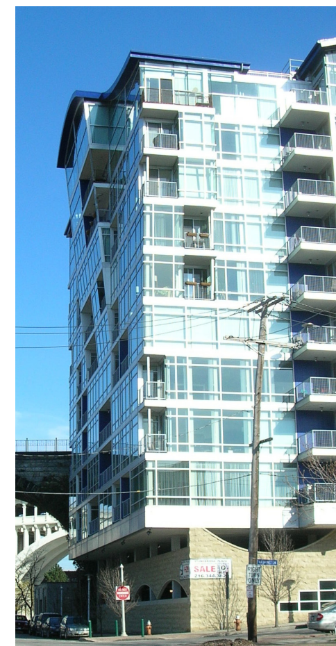
FIGURE III.31 - STONEBRIDGE FORMS A CONTEMPORARY BACKDROP FOR THE HISTORIC AREA TO THE WEST.
