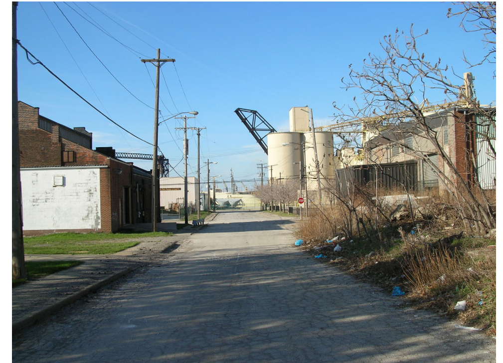
FIGURE III.34 - LOOKING NORTH DOWN HEMLOCK AVE.
