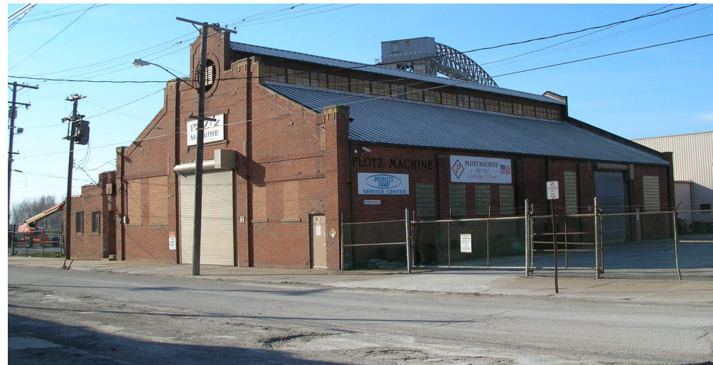
FIGURE III.28 - LOOKING NORTHWEST ALONG CENTER; BRICK STRUCTURE WITH GABLE ROOF, ROOF MONITOR AND CLERESTORY LIGHTING
