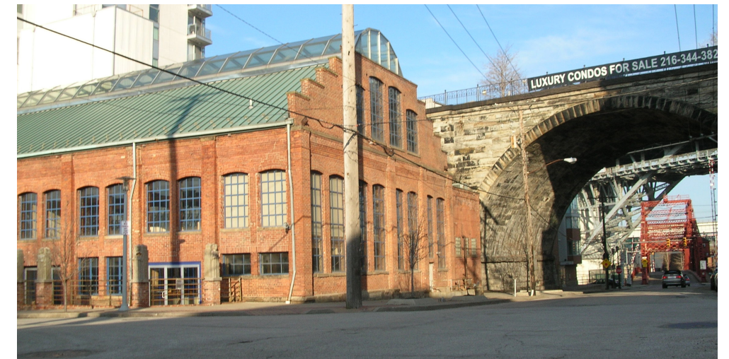
FIGURE III.24 - STONEBRIDGE AT CENTER STREET AND WASHINGTON AVENUE, WITH THE HISTORIC STONE SUPERIOR VIADUCT BEYOND.
