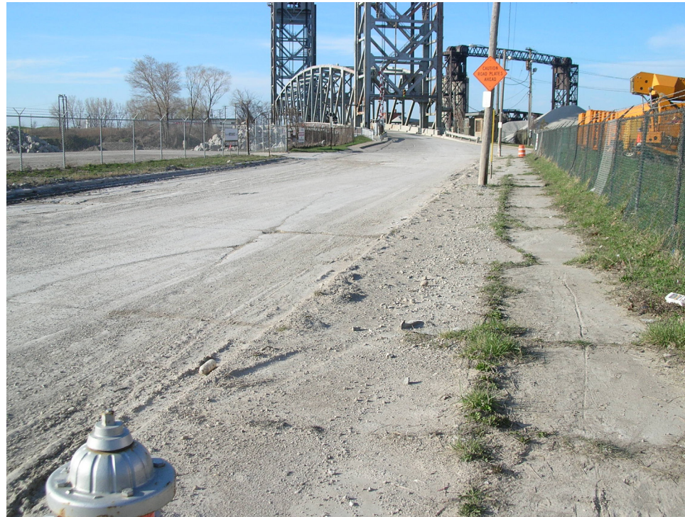
FIGURE III.33 - VISTA DOWN RIVER ROAD TOWARDS WILLOW STREET BRIDGE
