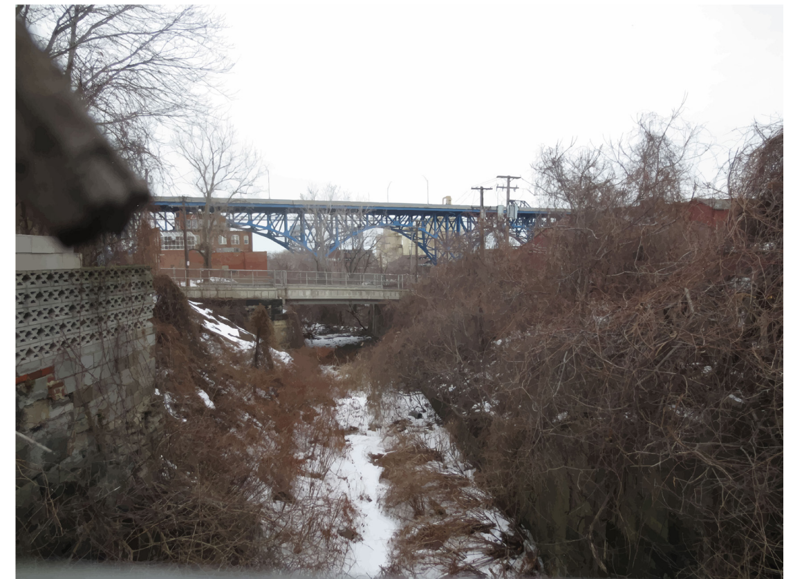
FIGURE III.16 - LAKE LINK TRAIL CORRIDOR BEFORE
