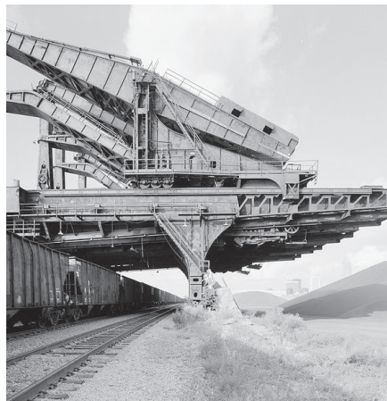
FIGURE I.1 - C&P ORE DOCK
