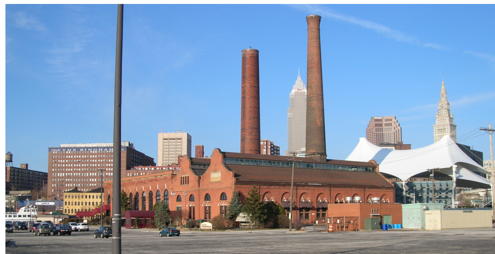
FIGURE III.29 - LOOKING NORTHEAST TOWARD NAUTICA, IN THE FORMER WEST SIDE POWERHOUSE, WITH THE DOWNTOWN CLEVELAND SKYLINE IN THE BACKGROUND.
