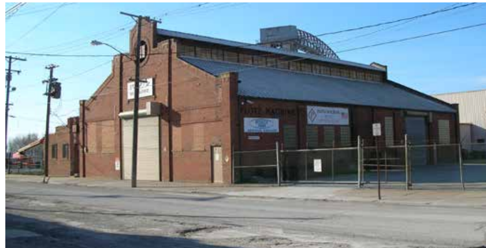
FIGURE III.28 - LOOKING NORTHWEST ALONG CENTER; BRICK STRUCTURE WITH GABLE ROOF, ROOF MONITOR AND CLERESTORY LIGHTING
