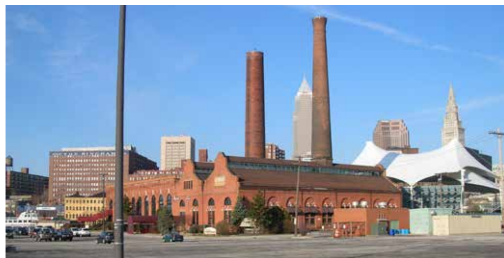
FIGURE III.29 - LOOKING NORTHEAST TOWARD NAUTICA, IN THE FORMER WEST SIDE POWERHOUSE, WITH THE DOWNTOWN CLEVELAND SKYLINE IN THE BACKGROUND.
