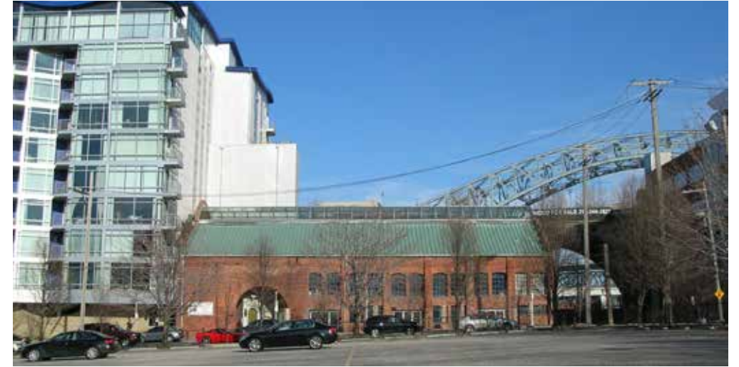
FIGURE III.30 - LOOKING EAST TOWARD STONEBRIDGE, SUPERIOR VIADUCT AND THE DETROIT SUPERIOR BRIDGE IN THE BACKGROUND.
