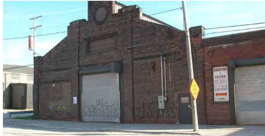
FIGURE III.27 - SOUTHWEST CORNER OF CENTER AND HEMLOCK; BRICK STRUCTURE WITH GABLE ROOF, ROOF MONITOR AND CLERESTORY LIGHTING.
