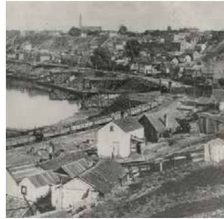
FIGURE I.2 - VIEW OF IRISHTOWN BEND
