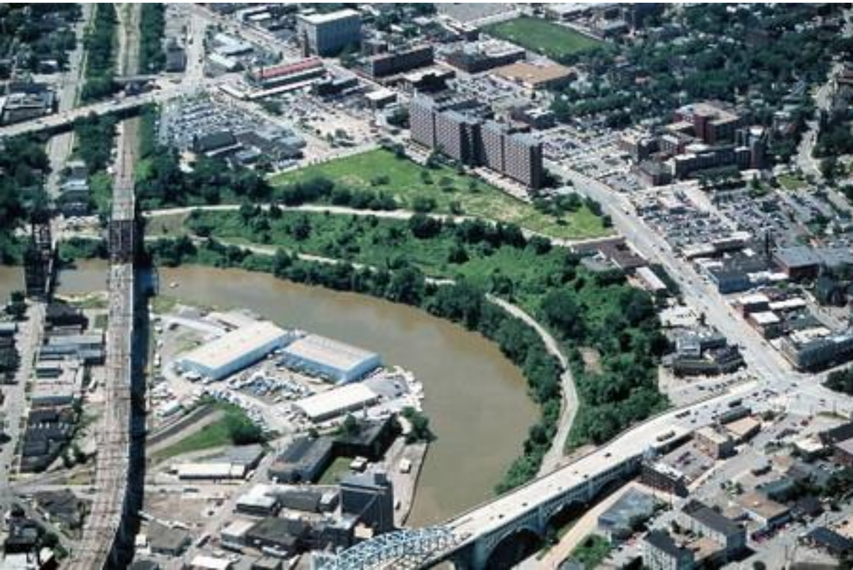
Source: Larry Hamel-Lambert/The Plain Dealer file. An aerial view taken in 2000 shows how the Cuyahoga River cuts a sharp curve below the geologically unstable Irishtown slope.
