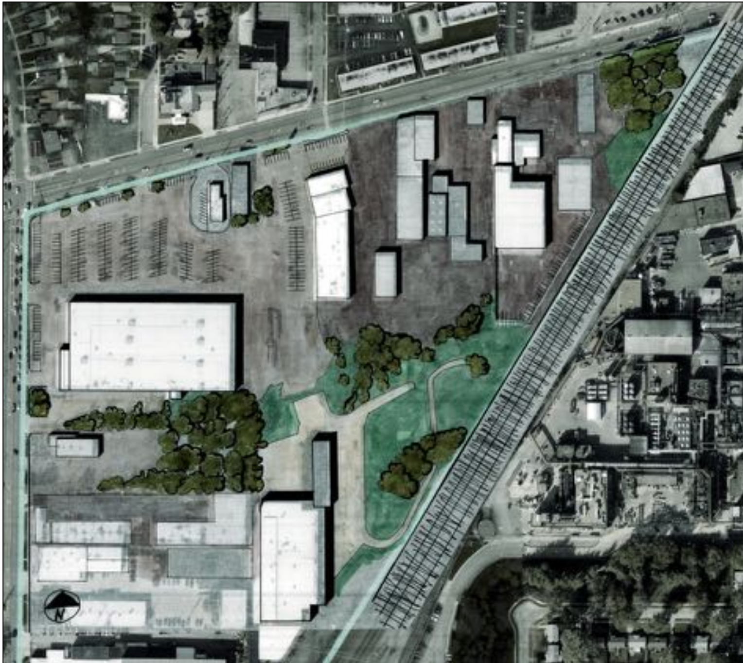
Figure 85. Existing Site Conditions (Viking Planning Group)
