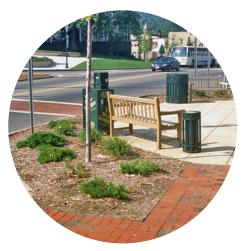
Curb bump outs can function as both stormwater capture and traffic calming elements (Source: SF Better Streets)
